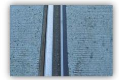
Figure 3 - Grooved rail with steel flangeway
