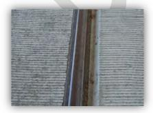
Figure 2 - Tee Rail with concrete flangeway
