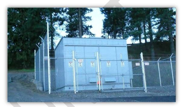
Figure 16 – Pre-fabricated substation (low-power) for the Portland Streetcar
