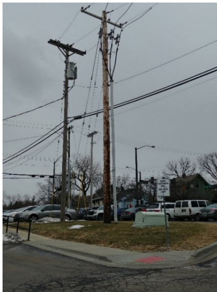
Figure 1: Potential Utility Conflicts at 51 st and Brookside Blvd.
